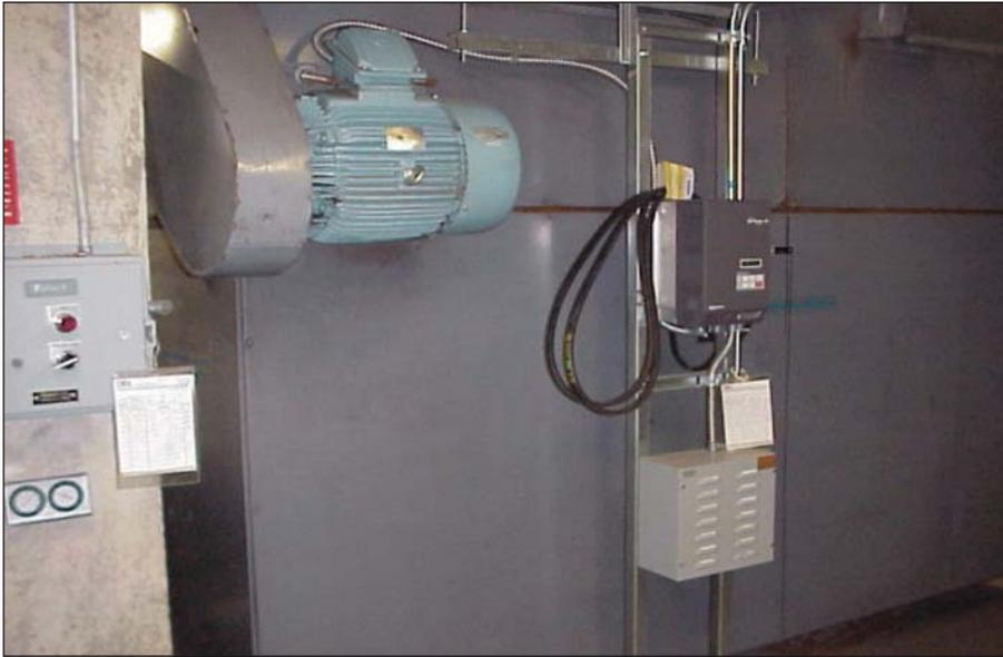
Figure 4. New fresh air supply fans
