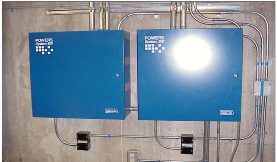
Figure 3. New building automation system
